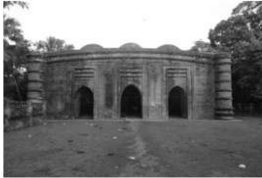
Fig.5 Facade of Nine-Domed Mosque,
