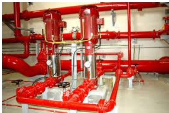
Sistem Hydrant (Pompa Kebakaran Jockey)
