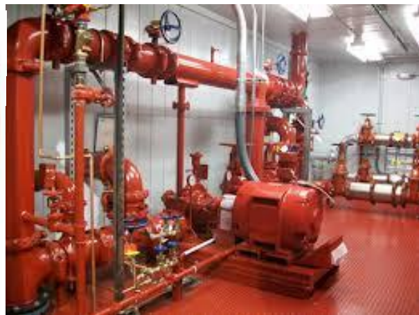
SISTEM HYDRANT (POMPA KEBAKARAN ELECTRIC)
