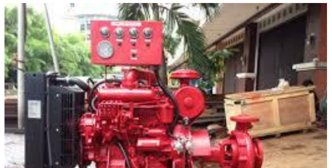
SISTEM HYDRANT (POMPA KEBAKARAN DIESEL)
