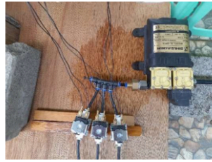
Figure 3.11 Garden solenoid installation
