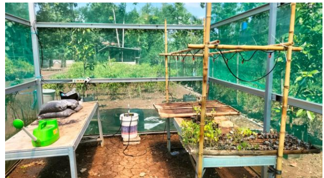
Figure 4 Automatic watering system for greenhouse .
