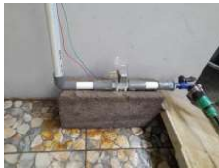
Gambar 4.12 Instalasi Main Valve (Q1)
